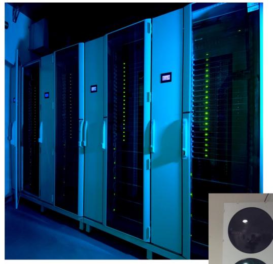
4 Racks, Rittal air/water cooling, 30 kW cooling capacity each
